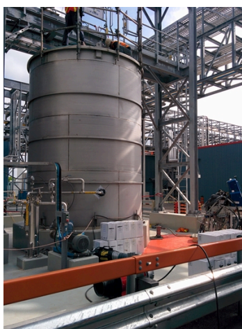
Tank after sand blasting.
