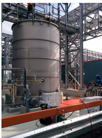
Tank after sand blasting.
