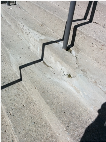
Cracks on stairs before repair.
