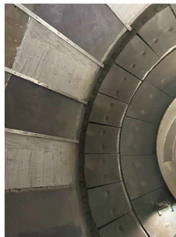
Close shot of the application in process.
