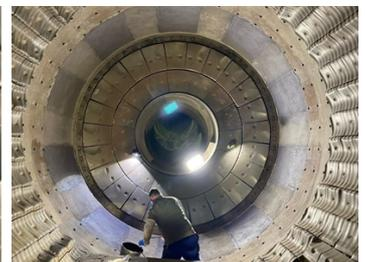
The damaged area half way covered with Belzona 1812 (Ceramic Carbide FP).
