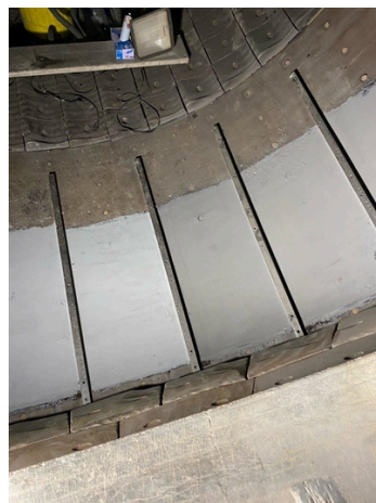
The damaged area repaired with Belzona 4111 (Magma-Quartz).
