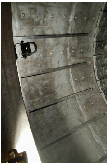
Tube mill grit blasted by the customer.
