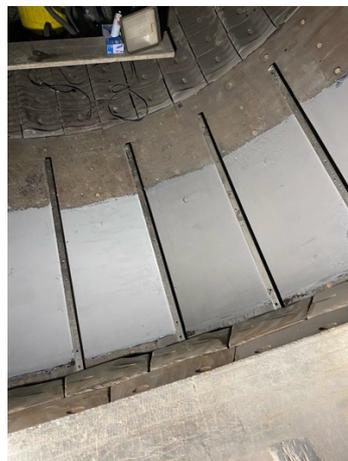
The damaged area repaired with Belzona 4111 (Magma-Quartz).
