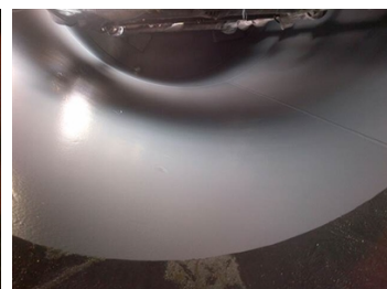
Lining application completed with Belzona 4311.
