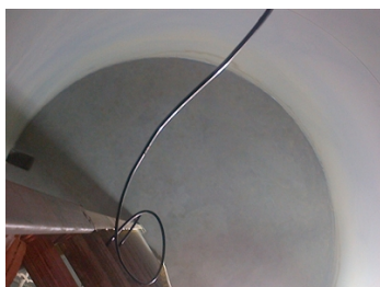
After abrasive blasting surface preparation
