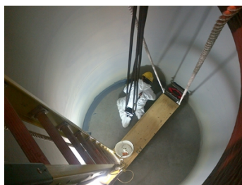
During stripe coating of Belzona 4311
