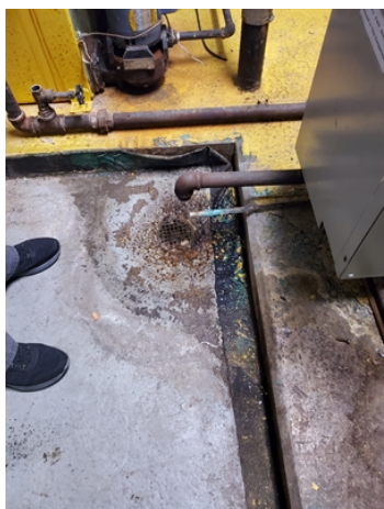
Drain condition before repair with Belzona
