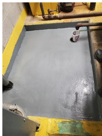
Final application of Belzona solution
