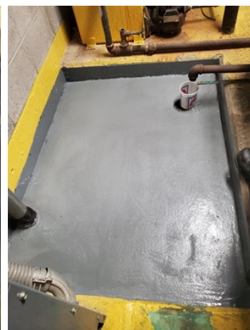
Final application of Belzona solution
