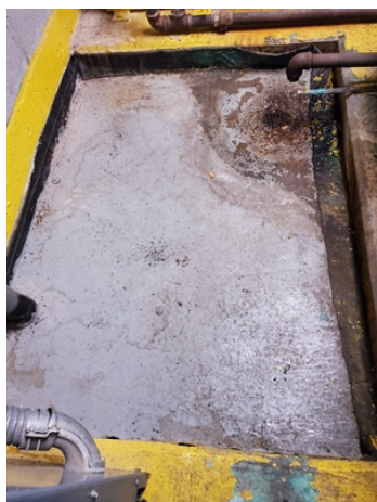
Drain condition before repair with Belzona
