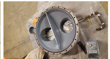
Protection completed with Belzona 1321.
