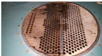
Tube sheet section damaged.
