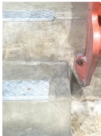
Savannah Civic Center Repaired with Belzona 4111.
