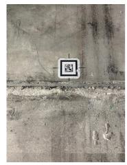
Close up of the damaged expansion joint. Most of the facility's expansion joints resembled this.
