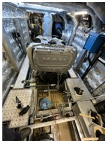
Ferrie engine room proved to be a difficult application due to confined space.
