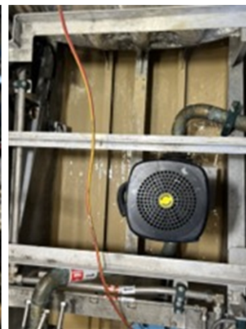
Belzona 5831 coated carried out successfully.
