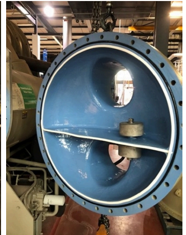
Completed coating on the end cover of the chiller unit.
