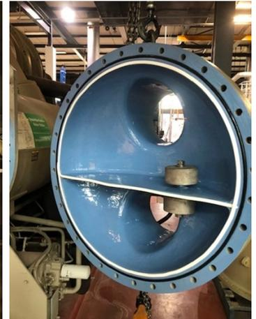
Completed coating on the end cover of the chiller unit.
