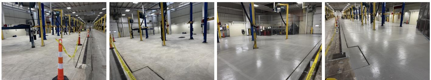
This building is being done in 4 sections. This area has been blast cleaned and is ready for Belzona 5231.
