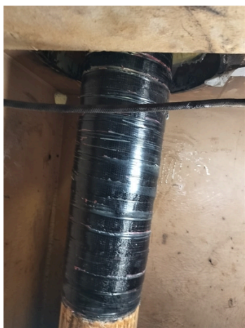
Pipe Section Two SuperWrap II Completed
