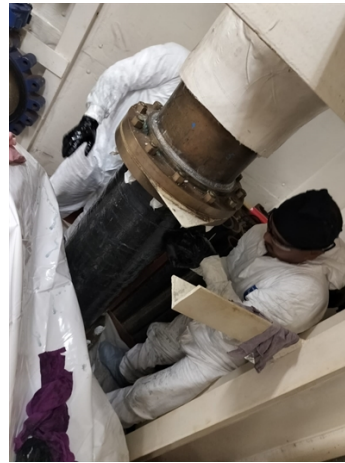
SuperWrap II being applied on the pipe section
