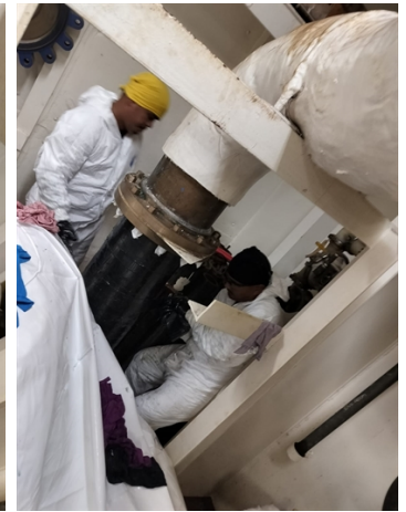
SuperWrap II pipe section being finished.
