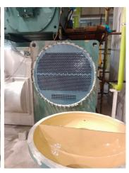
Belzona 5821 applied as 2 coat system to protect the tube and the end cover.
