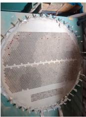
Work in progress, surface preparation with grit blast, rubber and plastic plug inserted.
