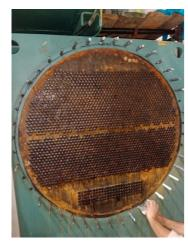
Picture taken during site visit noticed heavy corroded and damaged and measurements taken.
