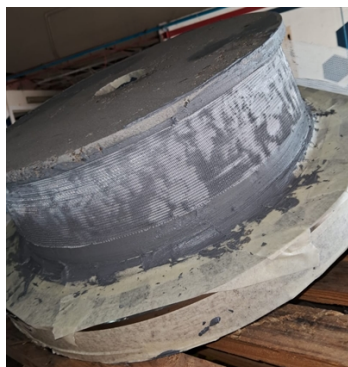
During the rebuilding works using Belzona 1121.
