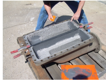
Division bar cast and cooler head being coated with Belzona 1311
