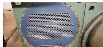
Tubesheet face before blasting and coating
