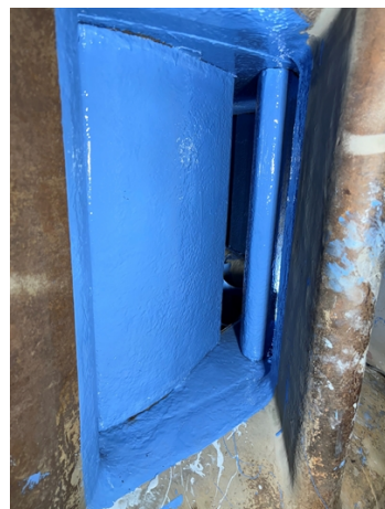
Completed with second coat of Belzona 1341 Blue
