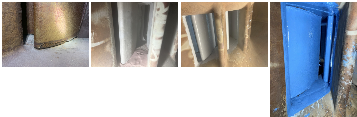
Existing condition of guide veins
