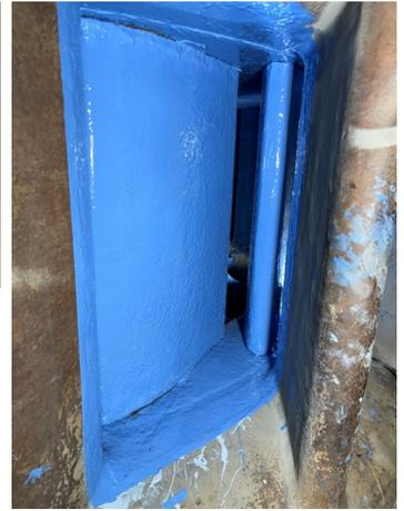
Completed with second coat of Belzona 1341 Blue
