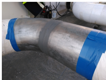
Surface preparation and weld seam rebuilt with Belzona 1212 E Metal
