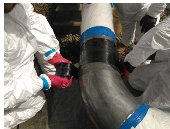
Application of Belzona 9381 Reinforcement Tape
