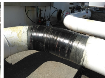
Super Wrap II repair completed
