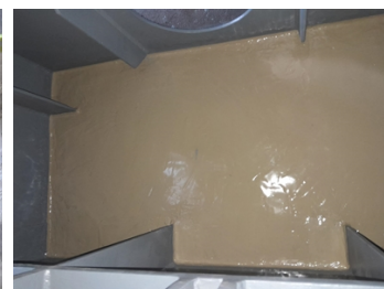
The rebuilt surface was overcoated with Belzona 5831 (ST-Barrier)
