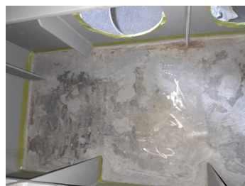
Surface preparation prior to the application of Belzona system
