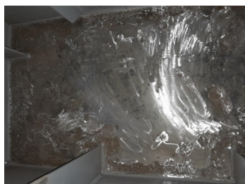
Surface preparation prior to the application of Belzona system
