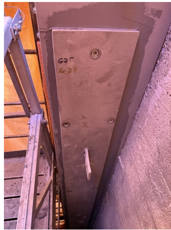
Structure after metal bonding with Belzona 1121.
