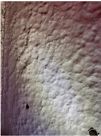
Structure before metal bonding.
