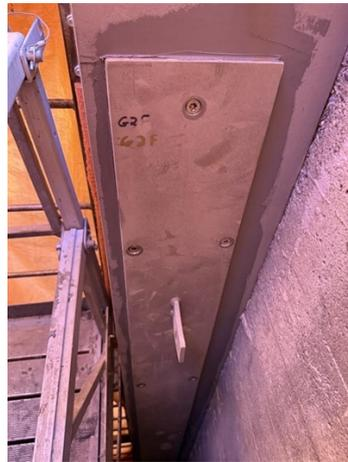
Structure after metal bonding with Belzona 1121.
