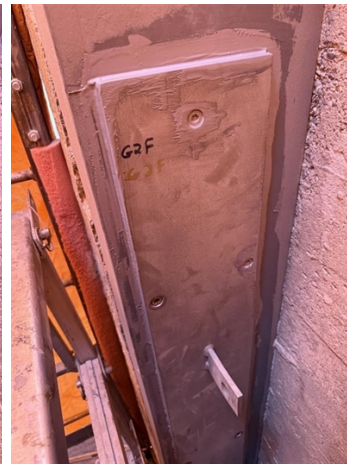
Perimeter of the bonded area coated with Belzona 5811.
