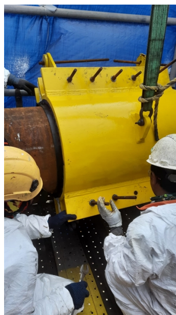
Clamping using a dummy pipe to compress the Neoprene Rubber sheet
