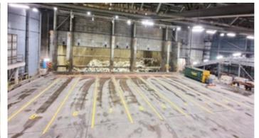
Completed Lorry Parking Bays and Numbers after application of Belzona 5231 Yellow
