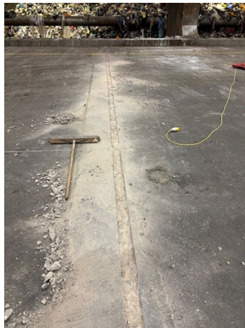
Bay Lanes Being Recessed Into Concrete
