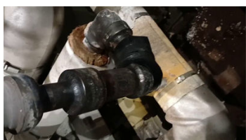
Leak arrested by Belzona 9611 and wrapped by tourniquet
