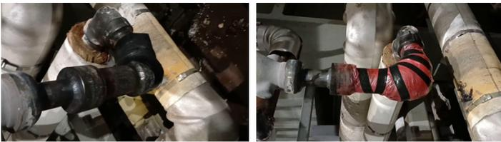
Leak arrested by Belzona 9611 and wrapped by torquiquet
