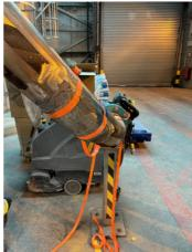
The steel patch now bonded into place over the hole and clamped with two strap clamps.
