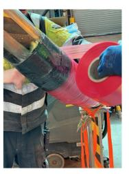
Belzona 1983 SuperWrap II has now been applied over the pipe elbow, covering the new patch and 200mm each side of this to give some structural Integrity back to the chute. Release film is being applied tightly to consolidate the application.
