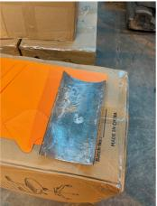
The Steel patch after surface preparation both sides, which is going to be bonded over the large elbow hole.
