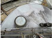
Belzona 4111 was trialed over the prepared areas and is set for future protection.
