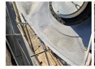
You can see the pooled water in the dip areas on the tank roof needing to be addressed.
