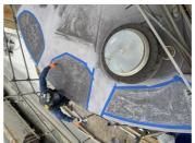
Belzona 4911 Conditioner is seen here be applied on top of the prepared steel.
