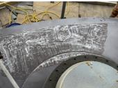
A diamond wheel grinder was used to achieve the appropriate profile on the low areas on the steel. The area was extended beyond the low points to be able to feather the product out and recreate a slope.
