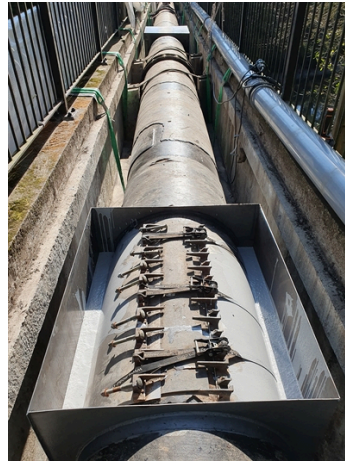
Steel frame placed into position 50% poured
