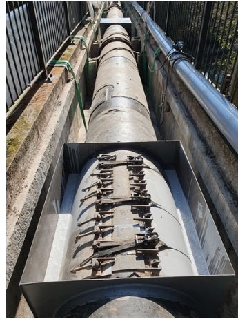
Steel frame placed into position 50% poured
