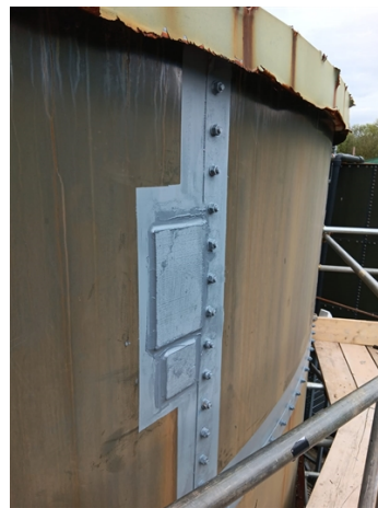
Composite plate bonded with Belzona 1111
