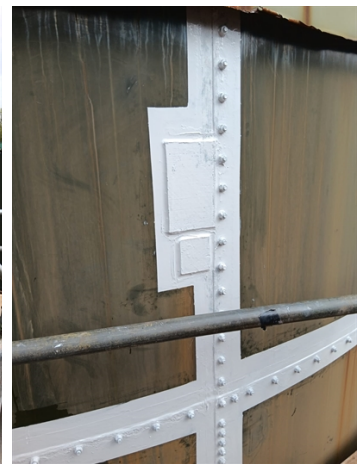
For added protection, all affected areas were then coated with Belzona 3131
