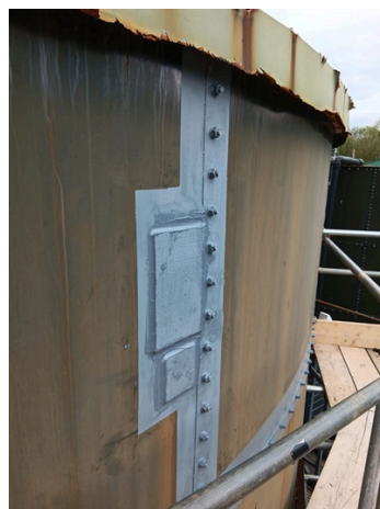
Composite plate bonded with Belzona 1111
