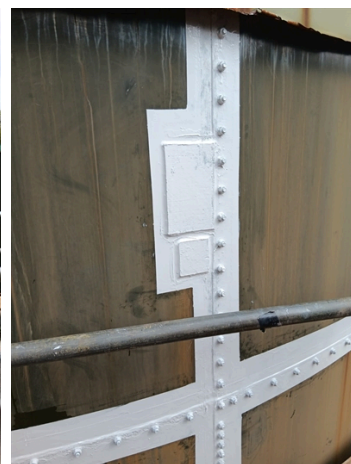
For added protection, all affected areas were then coated with Belzona 3131
