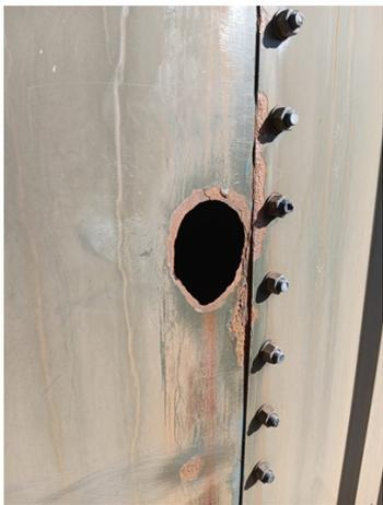
Through wall defects from internal chemical attack and environmental exposure
