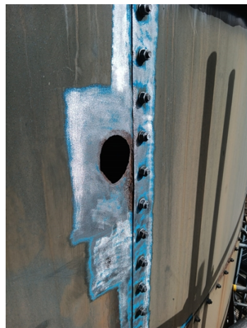
Surface area cleaned and prepared to minimum surface profile
