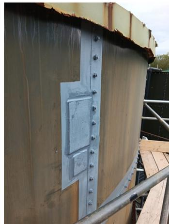
Composite plate bonded with Belzona 1111
