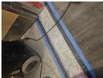
Removal of tripping hazard and surface preparation.
