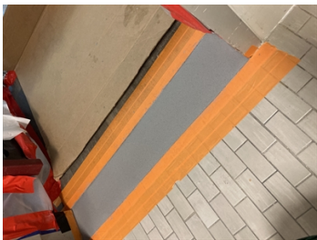
A new transition created with Belzona 4131.
