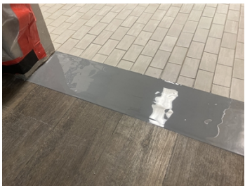
Belzona 4411 applied as topcoat.
