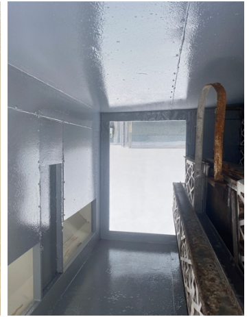
Air handler unit after application of final coat of Belzona 5811
