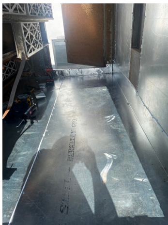
New metal was bonded using Belzona 1161
