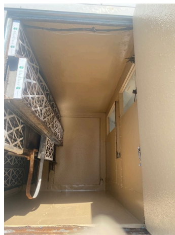
Air handler unit after application of Belzona 5831
