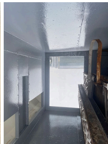
Air handler unit after application of final coat of Belzona 5811
