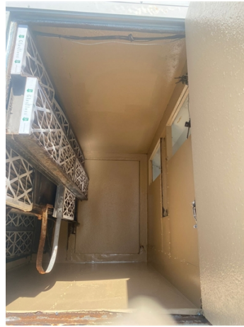
Air handler unit after application of Belzona 5831
