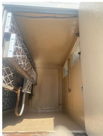
Air handler unit after application of Belzona 5831
