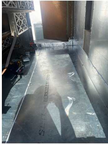
New metal was bonded using Belzona 1161
