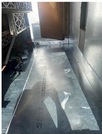
New metal was bonded using Belzona 1161
