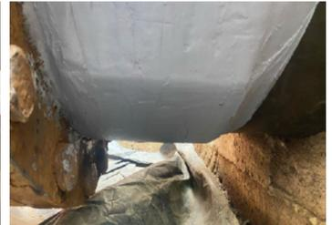
The entire area is wrapped with Belzona 1111 and Belzona 9341
