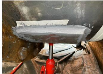
Plate is bonded over the defect area and clamped in place
