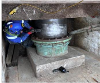
Surface area was prepared to minimum surface profile using power tools
