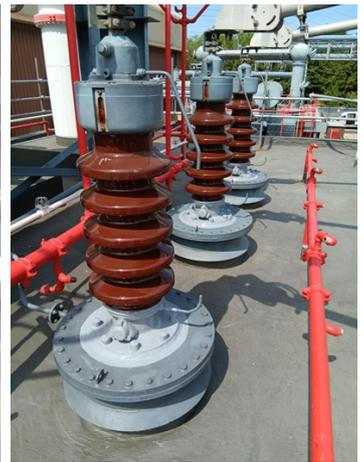
Encapsulation is complete and leak has been stemmed
