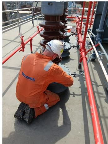
To complete application, a coating of Belzona 5831 is applied to encapsulate repair
