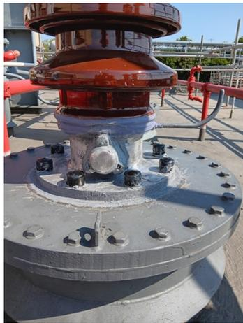
Existing paint removed and 1212 is applied
