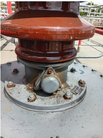
Bushing Flange Bases had been identified as leaking oil
