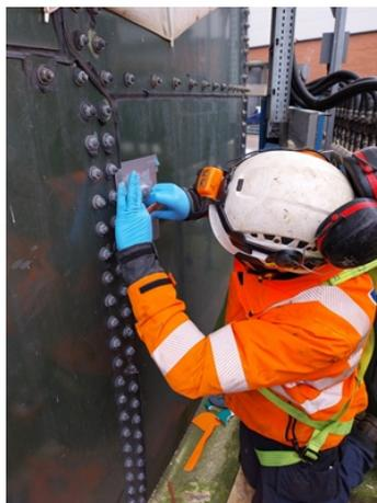
Carbon fibre plates were bonded using Belzona 1111
