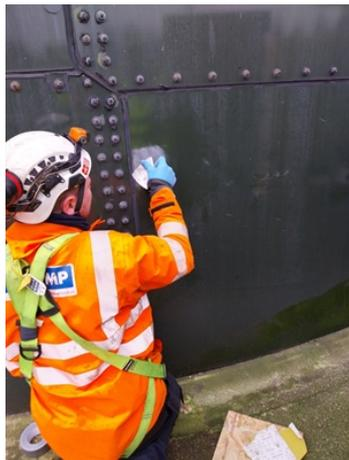
Several areas of external corrosion/damage were identified
