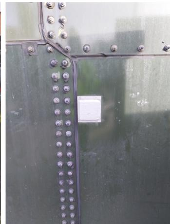
The solution ensures that no further corrosion can spread and weaken integrity of tank
