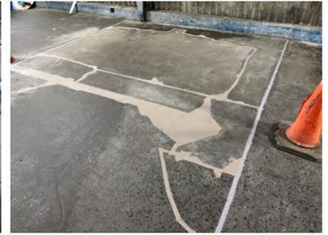
Completed Belzona 4131 areas & Belzona 4521 applied
