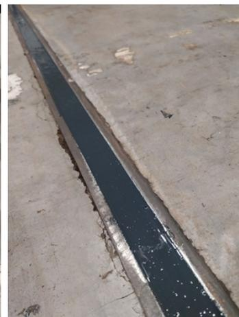
Expansion joints had separated over three decades, causing damage to forklifts operating in the area
