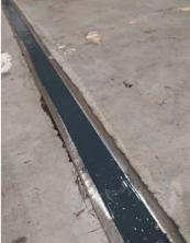
Expansion joints had separated The area is suitably prepared over three decades, causing damage to forklifts operating in to fill the area the area
