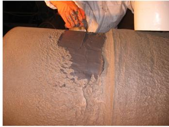
Belzona 1311 being applied to rebuild damaged areas
