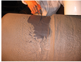
Belzona 1311 being applied to rebuild damaged areas
