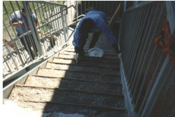
Cleaned and applying Belzona 4911 (TX-Conditioner)
