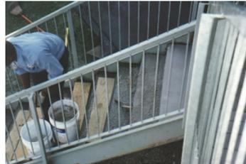
Belzona 4111 (Magma Quartz) being trowel applied
