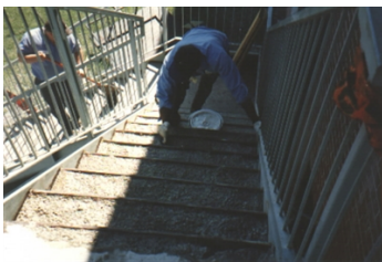
Cleaned and applying Belzona 4911 (TX-Conditioner)
