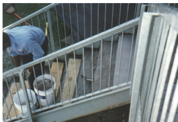
Belzona 4111 (Magma Quartz) being trowel applied
