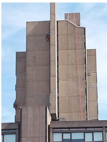
General view of the West face of the building, showing IRATA L3 Rope access engineers carrying out repair works with Belzona 4911 and Belzona 4141
