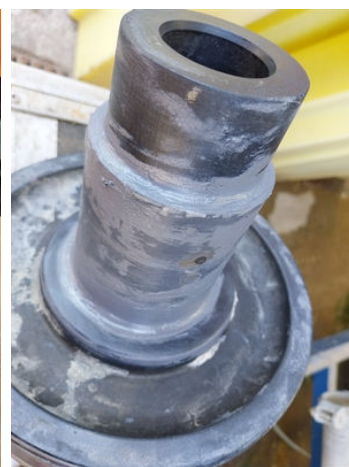
Both interfaces to the end cap fully sealed and ready to be refitted into the membrane housing
