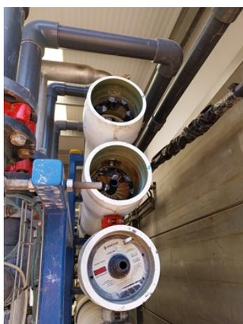
End cap receptor in RO Membrane housing
