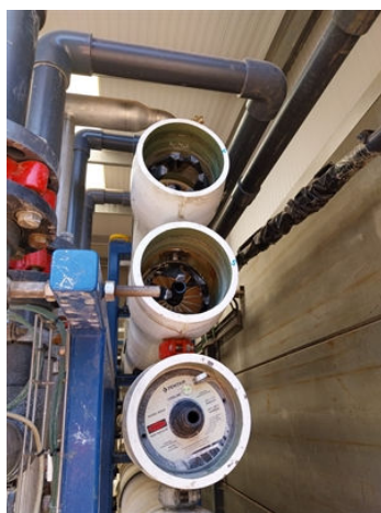
End cap receptor in RO Membrane housing
