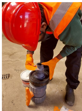
Applying Belzona 1212 to the 2 interfaces around the repair collar, previously glued, leading to a failed repair
