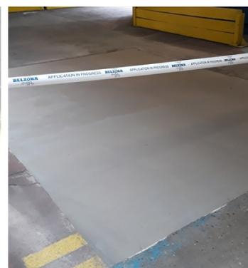
Area completely screeded at an average of 6mm using Belzona 4911 TX Conditioner and Belzona 4131 MagmaScreed
