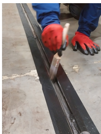
Joint taped and the application of Belzona 2911 Conditioner
