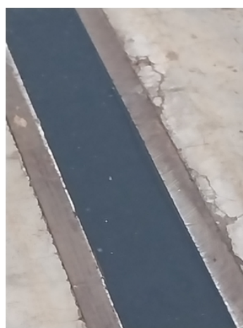
Expansion joint filled and tape removed
