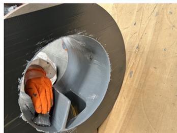
Two coats of Belzona 1321 are applied to end suction pumps
