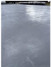
Before picture of the current coating that has delaminated in coating. Look how this coating 5815 with added aggregate for many areas.
