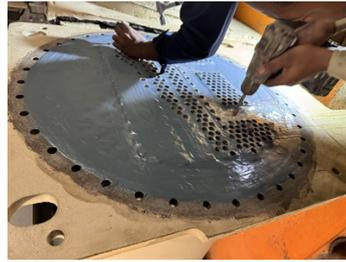
After (2) coats of Belzona 1321, the corks are then drilled out and the tubes are touched up.
