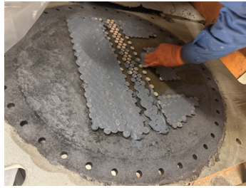
In Repair Process: Following Sandblasting, corks are placed and Belzona 1111 is used to rebuild low areas.
