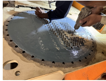
After (2) coats of Belzona 1321, the corks are then drilled out and the tubes are touched up.
