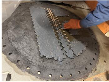
In Repair Process: Following Sandblasting, corks are placed and Belzona 1111 is used to rebuild low areas.
