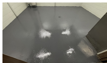
Completed (1) Coat of Belzona 5811 and (1) coat of Belzona 4311
