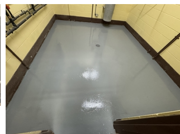
Completed (1) Coat of Belzona 5811 and (1) coat of Belzona 4311
