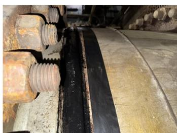
Completion Photo 2: Exterior View of Belzona 2111 applied to the Entirety of the Expansion Joint
