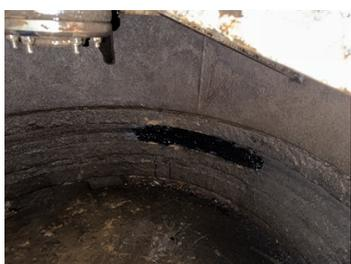
Completion Photo 1: Access into the Valve provided a chance to apply Belzona 2911, 2111 directly on the inside of where the leak had occurred. These products applied after preparing the steel+rubber.
