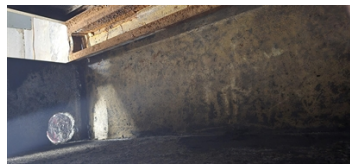
Inside look cooling unit pan before first coat
