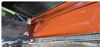
First coat of Belzona 5811 red
