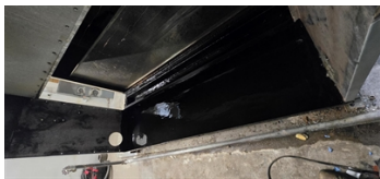
Second coat of Belzona 5811 black
