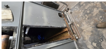
Outside look cooling unit pan before first coat
