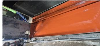
First coat of Belzona 5811 red
