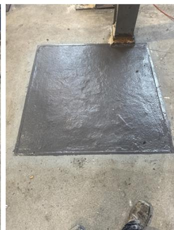
Repair completed with a final coat of Belzona 4311 to encapsulate the aggregate.
